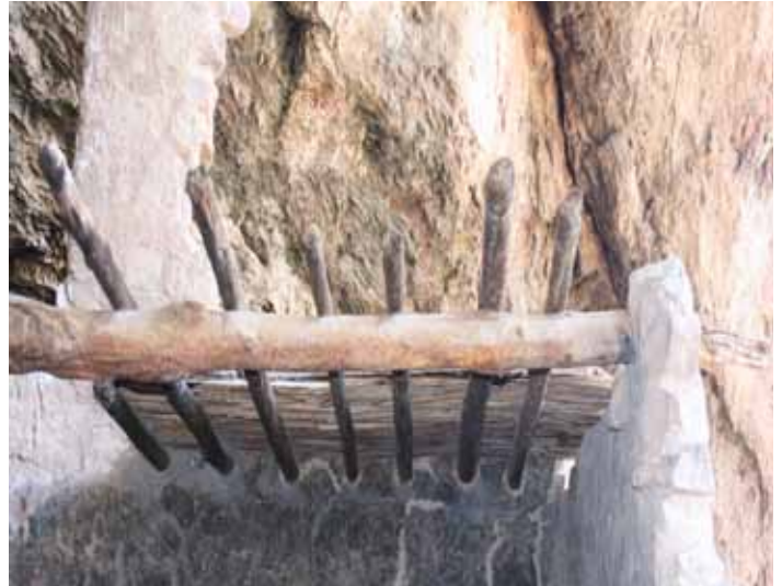
Roof beams in the Lower Cliff Dwelling at Tonto National Monument.
