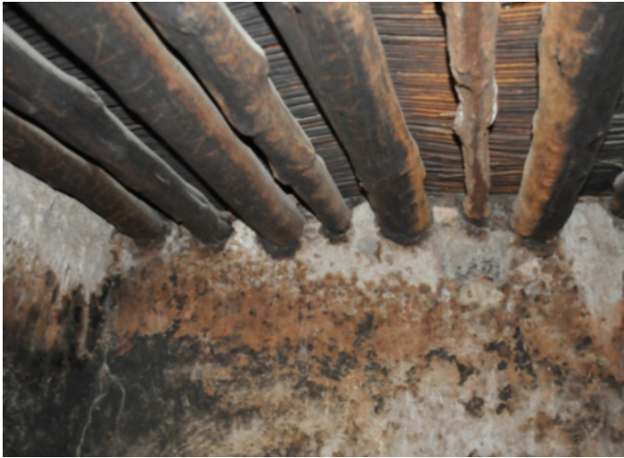
Healthy beams and a salt damaged beam in Room 1 (Level 4). The damaged beam also has significant beetle damage and severe wood defibration.
